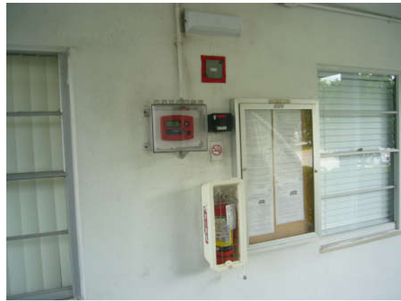
Upgraded Local Fire Alarm System & Controls
