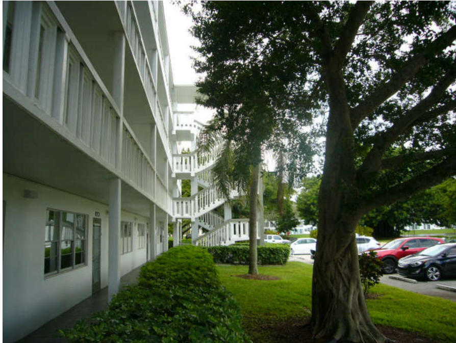
Stairwell with Balustrading
