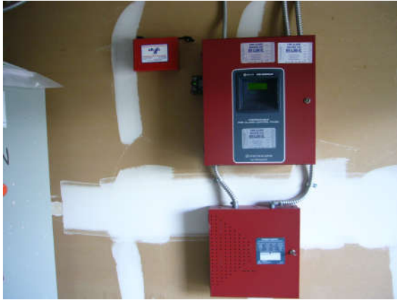
Upgraded Local Fire Alarm System & Controls
