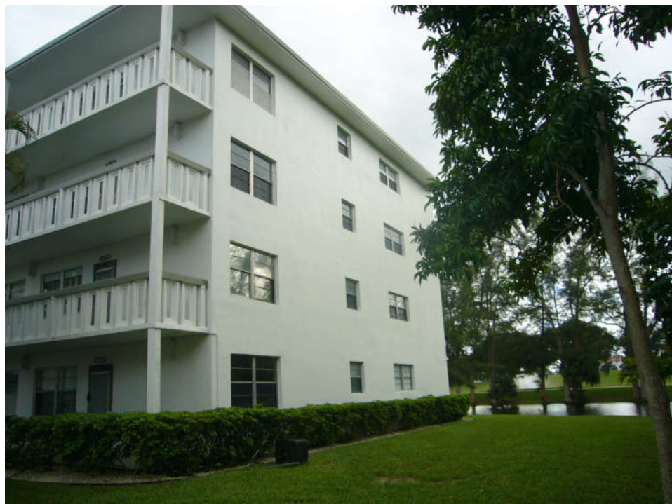
Side View of Building
