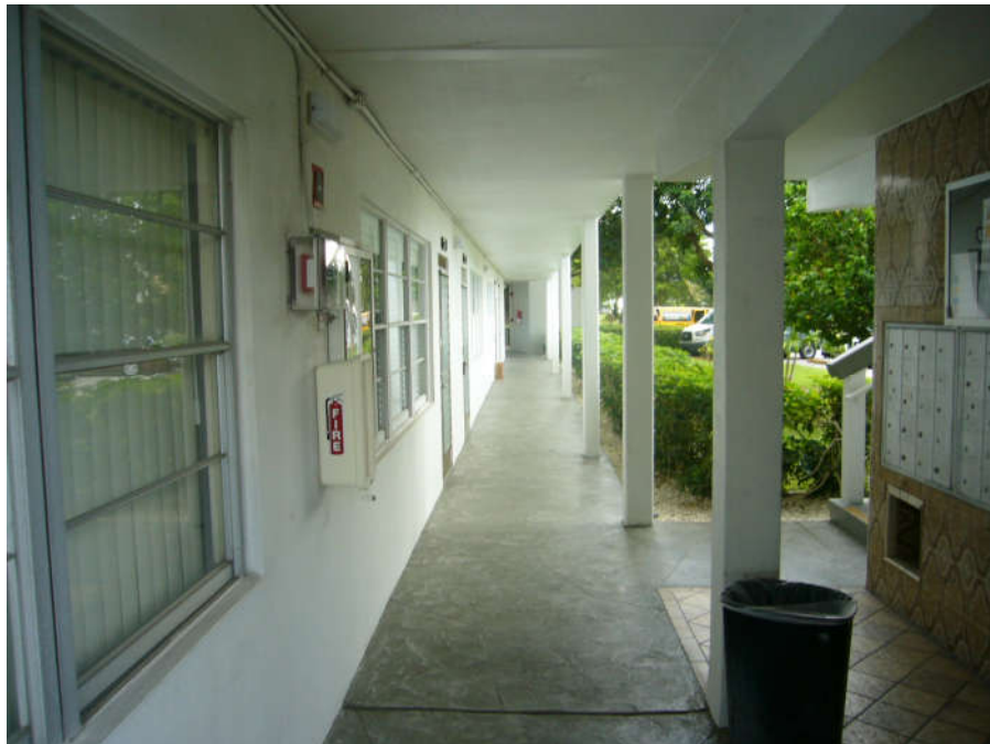
First Floor Entry Porch
