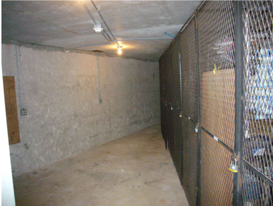
Typical Storage Facilities
