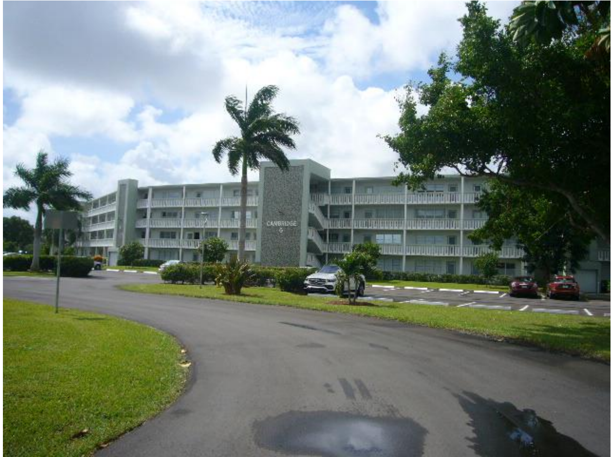
Front View of Building
