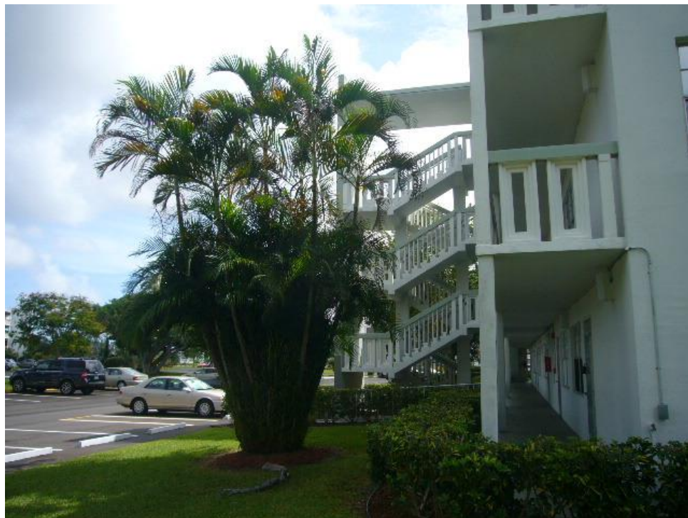
Stairwell with Balustrading
