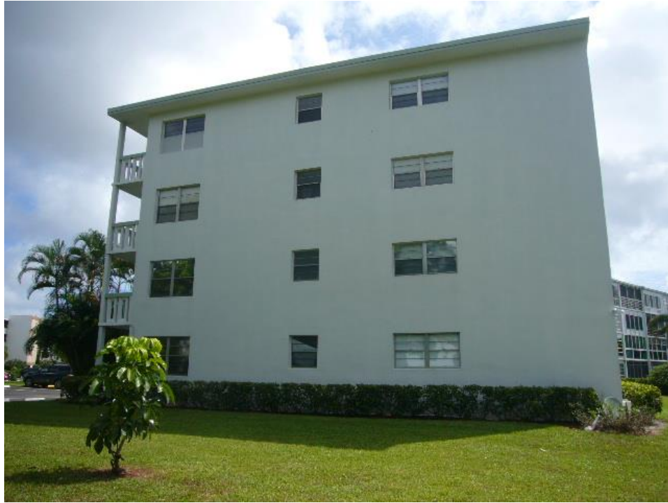
Side View of Building
